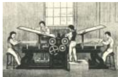
Putting-on and taking-off boys at a Taylor cylinder press - from Adams 1844
